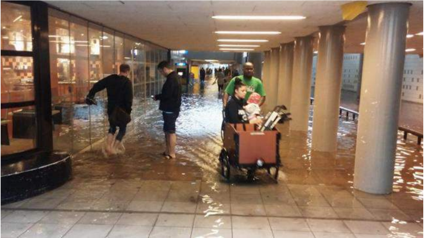
passenger tunnel at railway station
