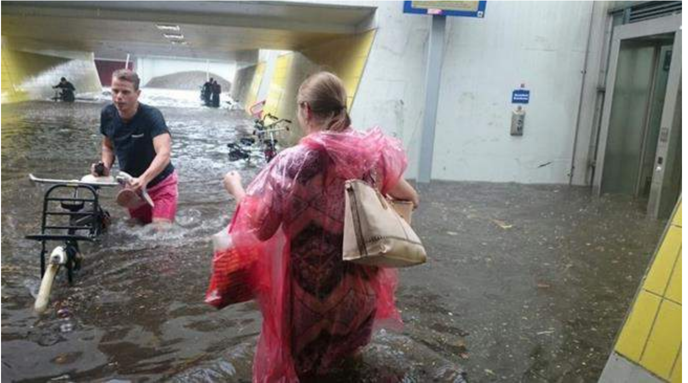
flooded passenger tunnel at railway station
